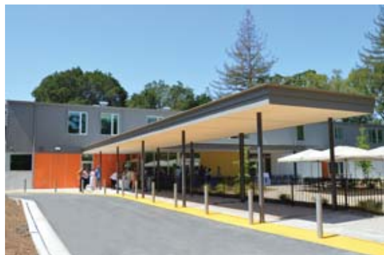
The newly renovated Las Trampas facility Photos courtesy Ian Craig
