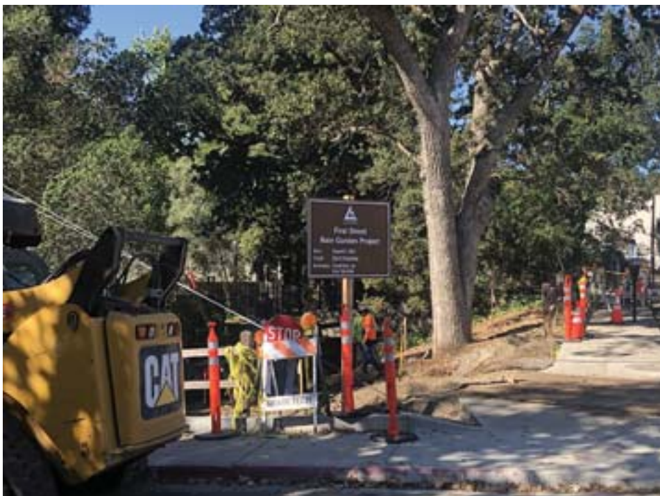
Rain Garden project work on Golden Gate Way in Lafayette.
