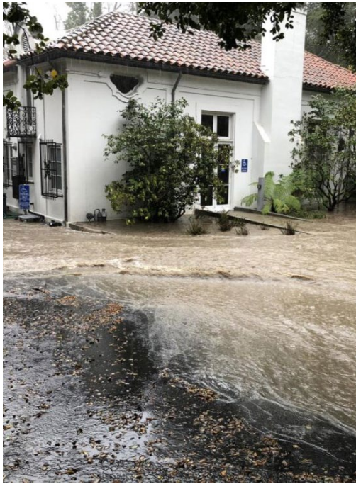
Flooding at Hacienda Park's Pavilion building Photo courtesy Moraga Public Works Department
