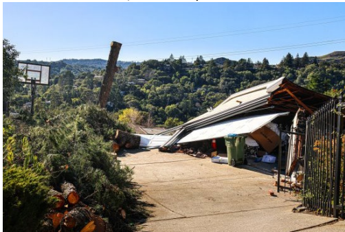
A collapsed garage sits at the end of this driveway on Cedar Lane. Photo Sora O'Doherty
