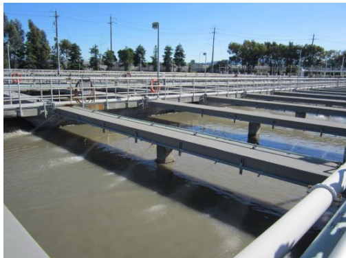
Primary Sedimentation process Photo Vera Kochan
