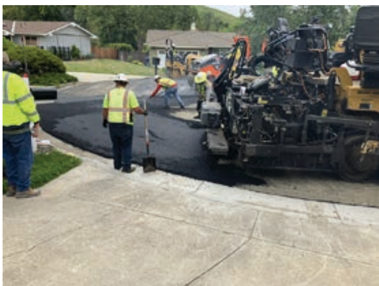
Photo courtesy Moraga Public Works
