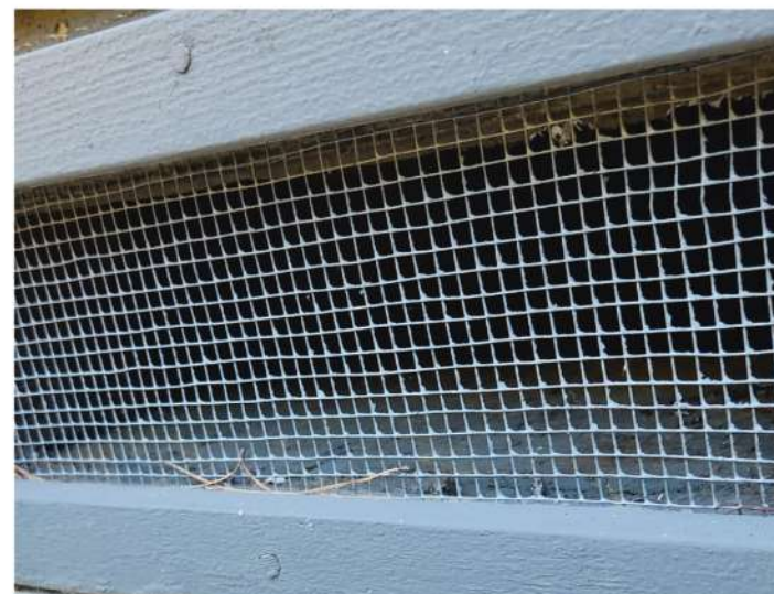
Foundation cover with 1/4 inch mesh
