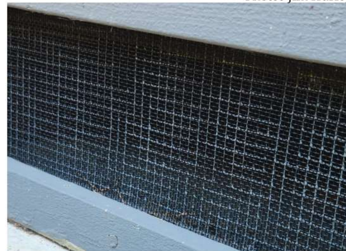
Foundation cover with additional 1/8 inch mesh
