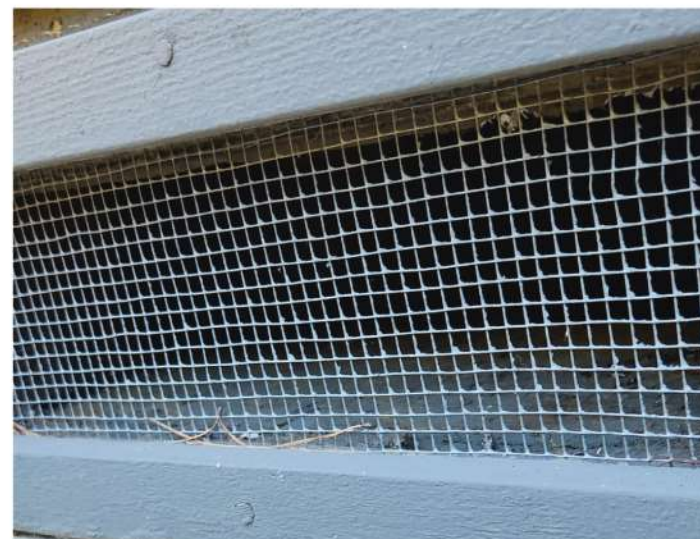
Foundation cover with 1/4 inch mesh
