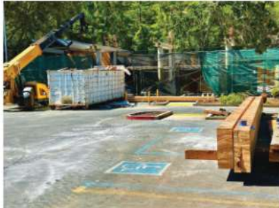
Construction has begun on the transformation of the old Bank of America building in downtown Orinda.
