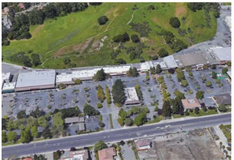
Aerial of Rheem Valley shopping area.
